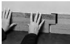
Install next tile as shown.
