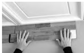
Moving left to right, use overlap notches to abut tiles, just as you would in a backsplash installation.
