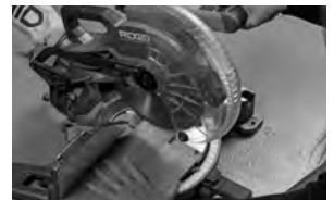
Cut away the notch with a miter saw.
