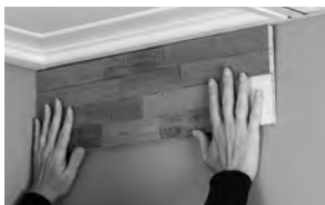
Beginning from inside corner on left, place the first tile.
