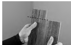
Cut away the notch with a miter saw.
