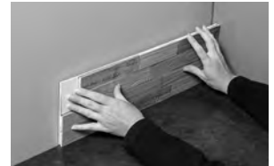
Beginning from inside corner on right, place the first tile.
