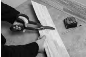
Cutting a straight cut with a snip
