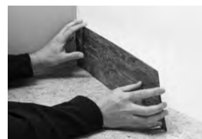
1) Place the first tile. Angle side or top of tile away from wall until you are sure of placement. Use the counter top as a guide as you move it into place.
