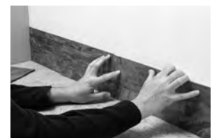
2) Leave adhesive backing on to "dry fit" the next piece throughout the entire installation. If you are satisfied with the dry fit, remove liner and apply the next tile the same way you did the first one.
