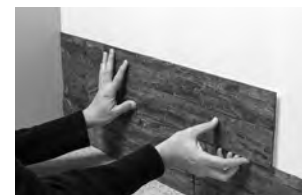
4) Carefully tip it up into place so it butts the last tile, then carefully install the tile while making sure the bottom edge is fitting tightly against the lower tile.
