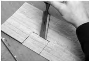
Cutting the inside edge with chisel
