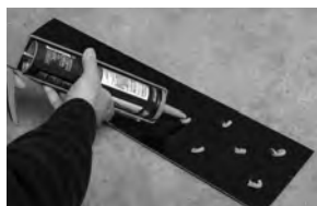
Method 2 - Using high-quality polyurethane construction adhesive
