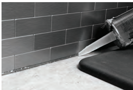
Caulking the counter top seam
