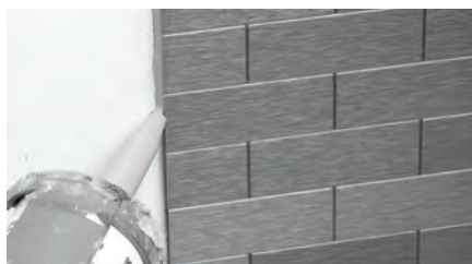
Finishing option 2: Caulking outside edges
