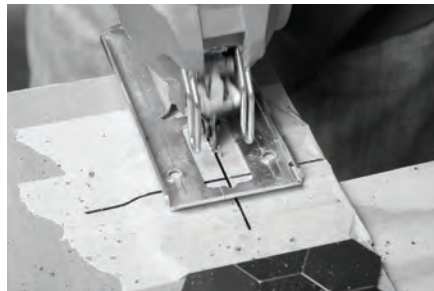
Cut the tile using the recommended cutting tools
