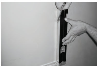
Mark horizontal and vertical reference points
