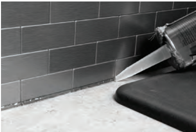
Caulking the countertop seam
